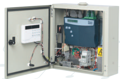
Squirrel 2020 in an electrical enclosure
